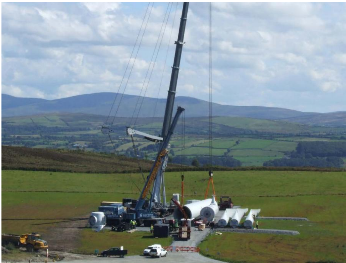
Plate 4.4: Wind Turbine Erection
