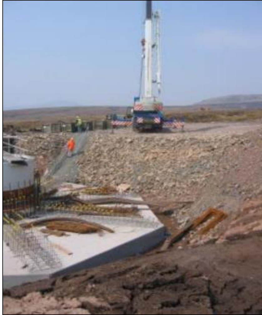
Plate 4.2: Turbine foundation under construction with adjoining crane pad 3
