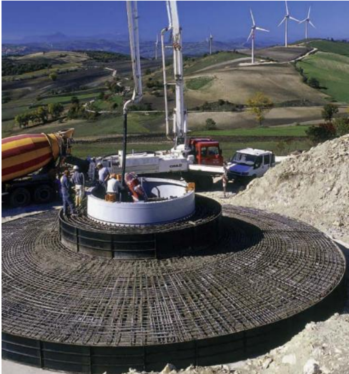
Plate 4.3: Wind Turbine Foundation
