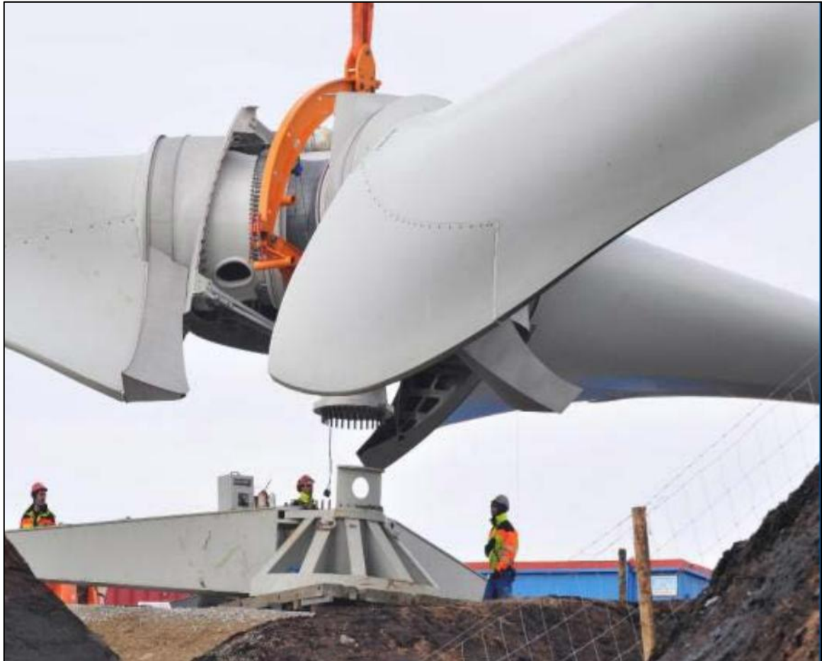
Plate 4.5: Assembly of wind turbine blades
