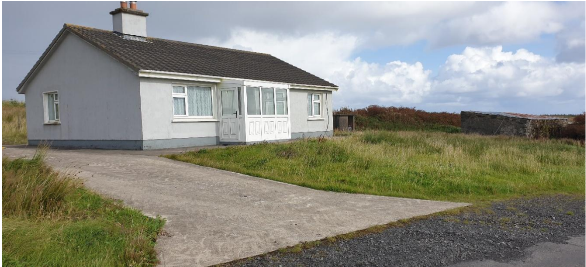
Plate 4.1: Proposed Existing Residential Site to be Converted to an Operations Building
